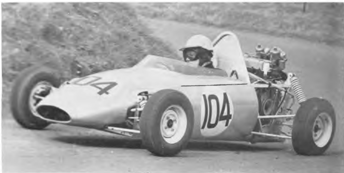
Alan Staniforth spent last Winter brewing up a very novel single-seater powered by a rear mounted Mini unit. Jeff Binns took this picture of the "Terrapin Min" on one of its first outings of the season at Castle Howard. Subsequent development has included the substitution of the hydraulic gear linkage with a mechanical system and the nakedness of the rear has been clothed.
