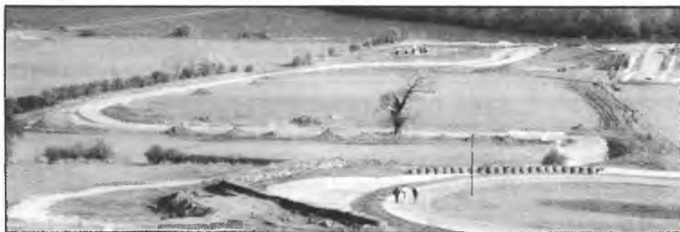
A view of the new track under construction.
