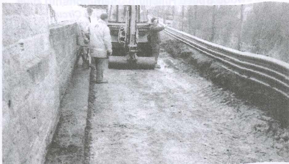
Scraping the road by the Farmhouse
